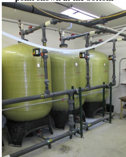
three of the four filter tanks
